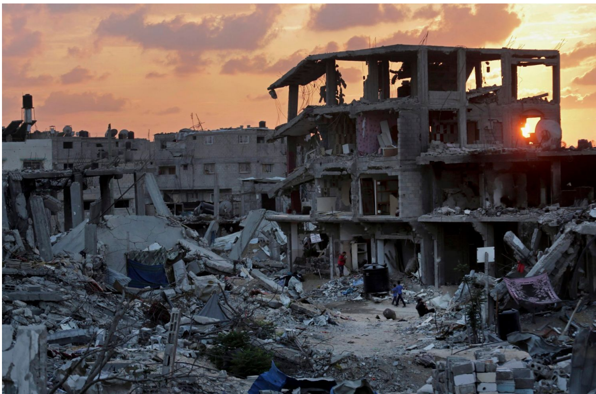
Palestinians walk during the sunset between the rubble of their destroyed building in Shijaiyah neighborhood of Gaza City in the northern Gaza Strip, Sunday, Oct. 12, 2014.
